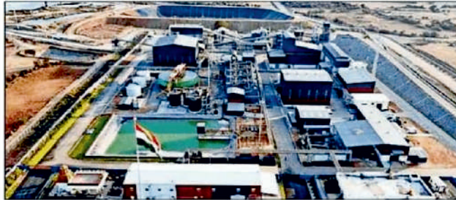
Aerial view of the project in Jonnagiri, AP. At peak capacity, it is expected to produce up to 1,000 kg of refined gold annually over next 15 years
